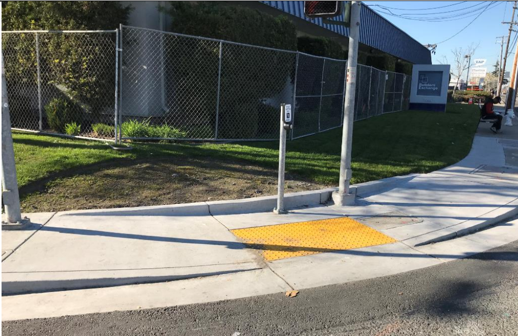
COMPLETED ACCESSIBLE CURB RAMP WITH RELOCATED PEDESTRIAN PUSH BUTTON
