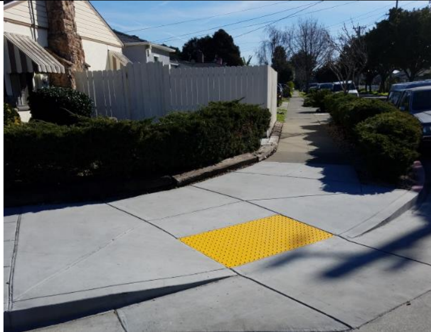
COMPLETED ACCESSIBLE CURB RAMP
